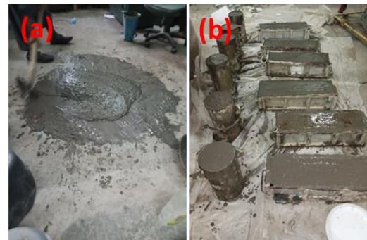
Figure 2 Mixing & Casting of SCGC (a. Mixing of SCGC, b. Casting of SCGC)
